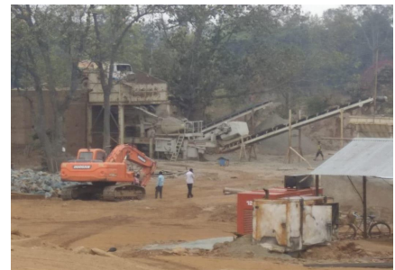
Crossing of hard rock of Deo Spillway
